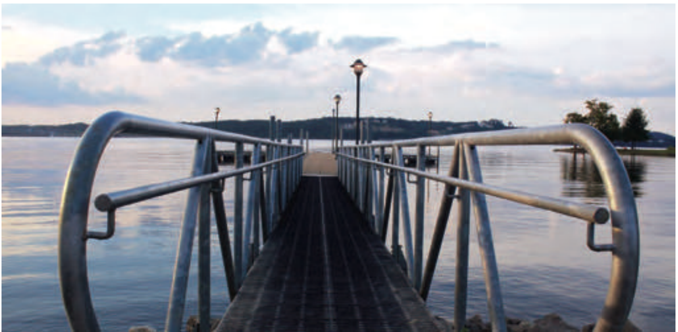
Pickwick Landing State Park in Tennessee: Not every bridge leads to somewhere but each and every one deserves a look.
